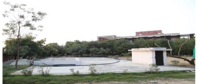
A Sewage Treatment Plant (STP) of 40 Cu. M. per day is used for wastewater treatment and reuse. Grey water is treated on the campus and used for the gardens.
