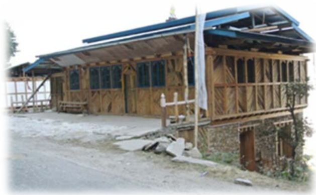
Temporary lease at Yadi, Monggar with permanent structure.
