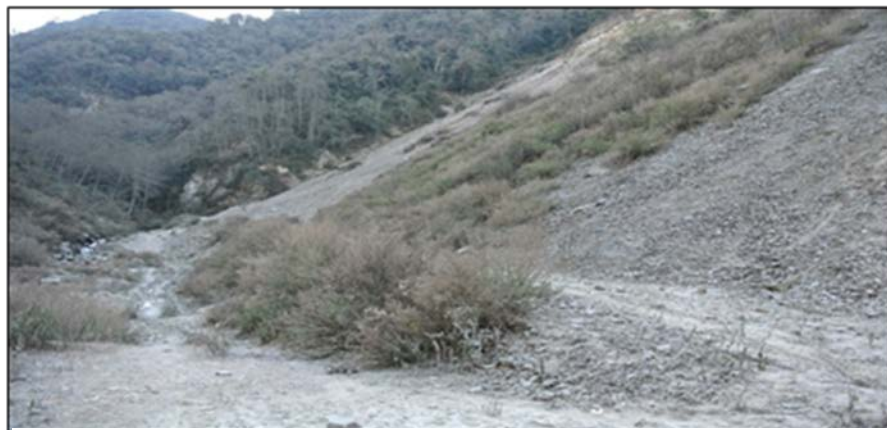
Design without benches at Lumjasam Stone Quarry
