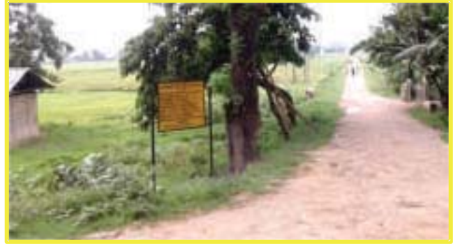
Electrification under RGGVY inside 2nd addition area
