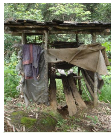
Hanging Toilet in Barilum, Kabjisa, Punakha.
