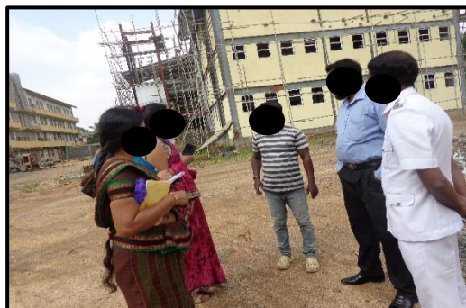
New building being built – Polonnaruwa Hospital
