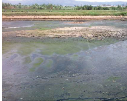
Sections of the Jinja ponds filled with sludge with evidence of channelled flow of the sewage.
