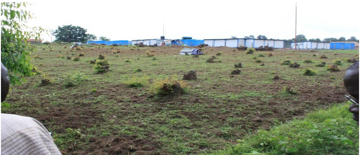
Picture 29 showing installations covering an approximate area of 3 ha claimed to be a project of Veterans in Arua CFR.
