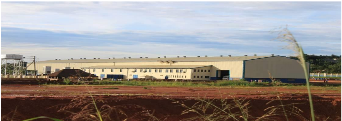
Cpt 12 of Namanve CFR: Newly constructed Roofing factory in Cpt 12.
