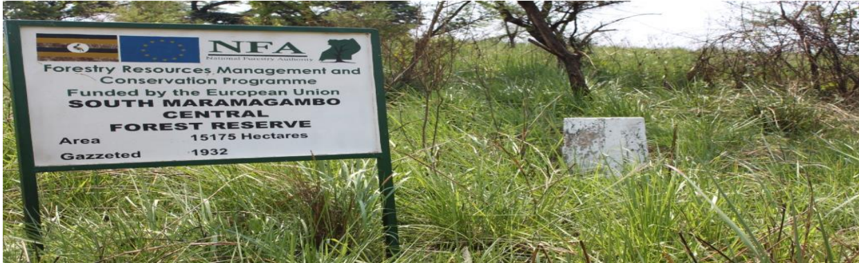
Conspicuous concrete pillar (Beacon) used for marking the forest boundaries in South Maramagambo CFR. This is desired demarcation feature to be used in un-clear forest boundaries by NFA. GPSC-N082°31'47" E993°52'38"
