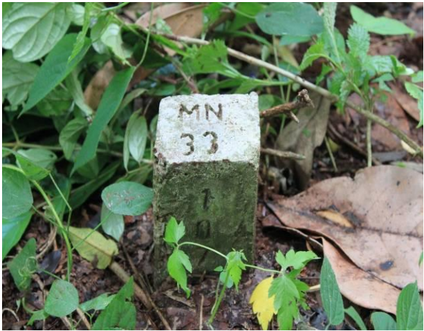
Corner Cairn in Mabira CFRs uncovered on inspection
