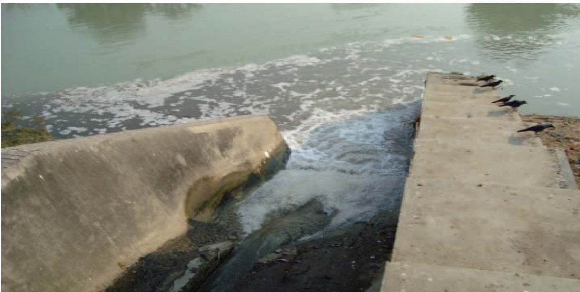
Untreated sewage flowing into Ganga in Haridwar
