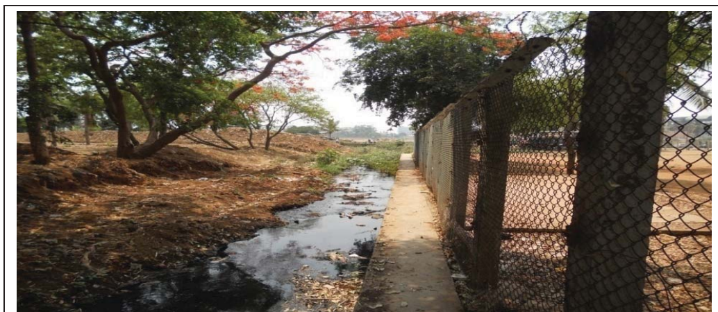
Dasarahalli Lake main drain (inlet 1 of the lake) receives all the effluents from Peenya Industrial area as evident from the thick viscous black water flowing in the drain
