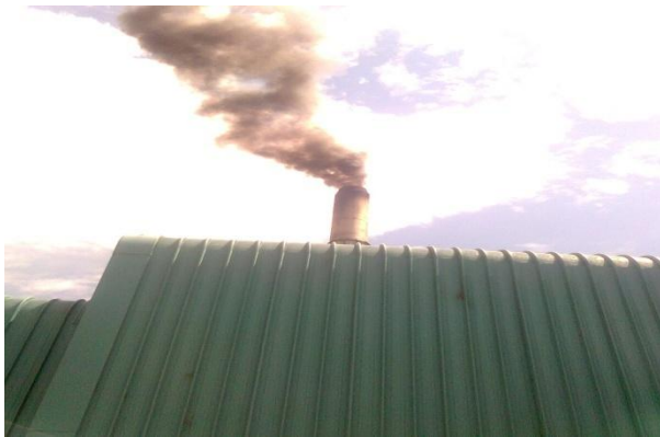
Smoke emitting from the Chimney
