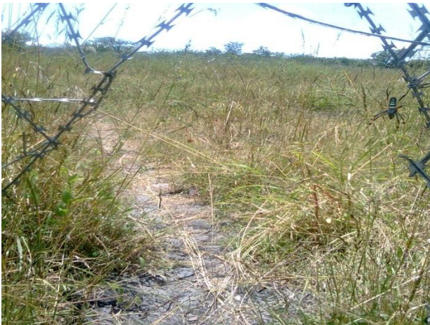
One of the Openings on the Landfill Fence
