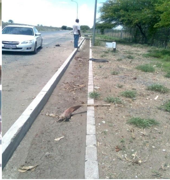
The designated Area for Washing Tyres
