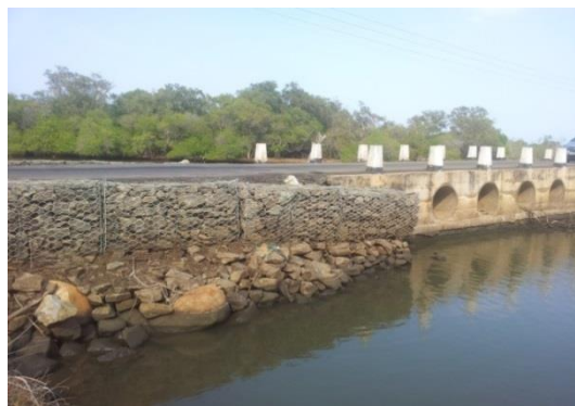
( The bridge that has been an obstacle to the sand transportation)
