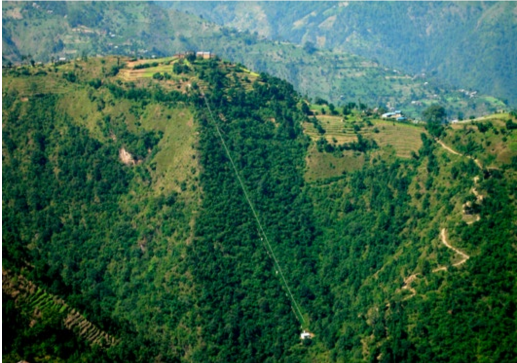
A remote village in Nepal is supplied with electricity from a micro power plant built by a Norwegian-supported programme. The programme has helped over 400,000 households gain access to electricity from solar or micro power plants.
