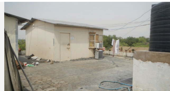
Temporary accommodation of NDRF headquarters created at roof top of Civil Defence Secretariat Building
