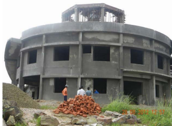
Under construction building for S-Band DWR at Cherrapunji
