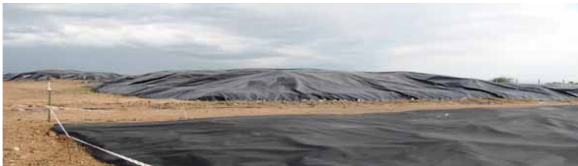
Picture 2: Showing a properly covered Pit at Kisinja WCA
