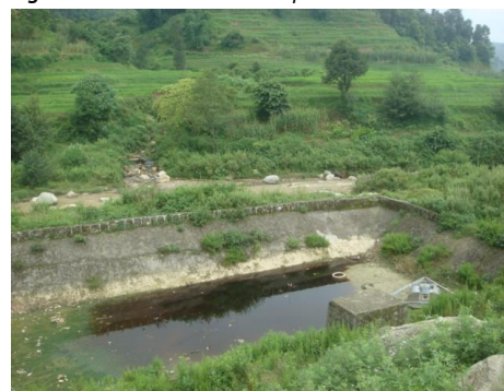
Figure 7: Leachate treatment pond in Sisdol
