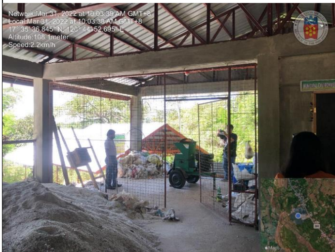
Enclosed area for waste processing of unsellable bottles using crusher/pulverizer equipment
