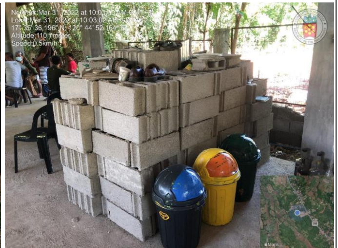
Designated area for finished Concrete Hollow Blocks (CHBs) made from pulverized unsellable bottles mixed with concrete
