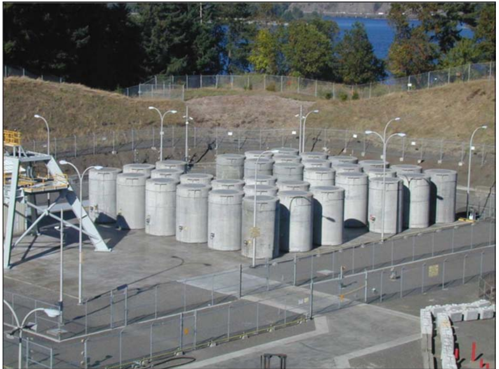
Figure 6: Spent Fuel in Dry Storage
